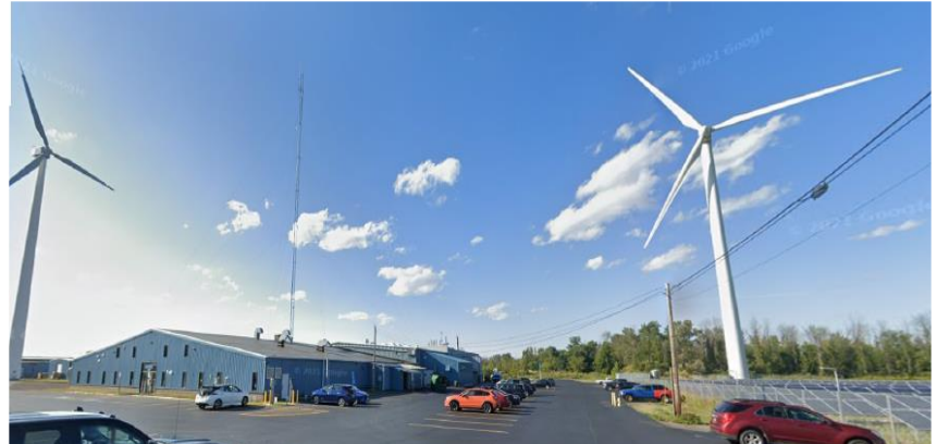
HARBEC Manufacturing Facility and Wind Turbines
