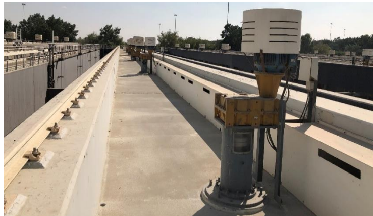
Installation of VFD's at the aerators at Al Mafraq STP
