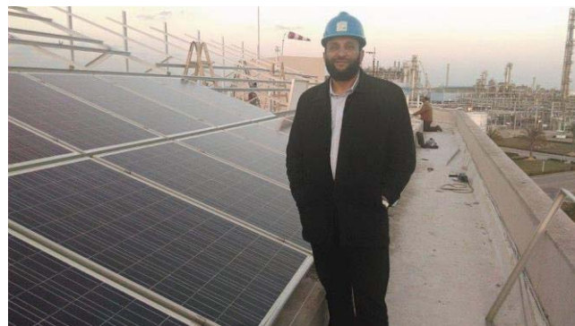
During the installation of SIDPEC solar station March 2015
