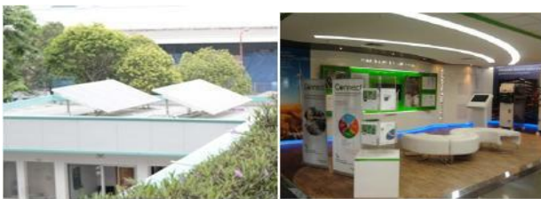
Installation of solar panel to support the energy in the lobby show room
