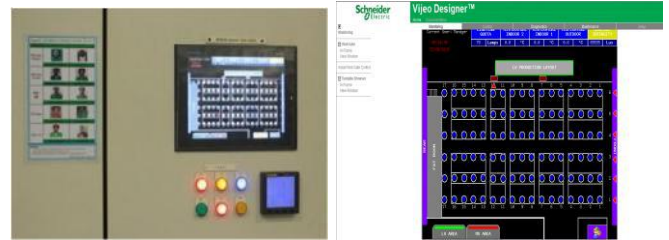
Install of Production Lighting control system.
