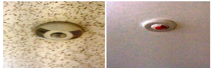
Install sensor movement in all meeting & toilet room.
