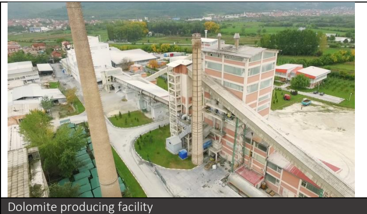
Dolomite producing facility
