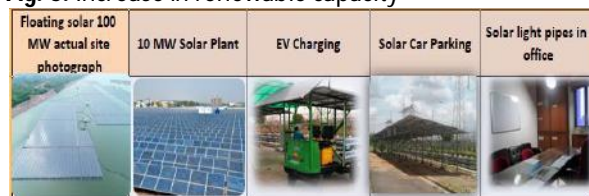
RE Power set up at NTPC Ramagundam
