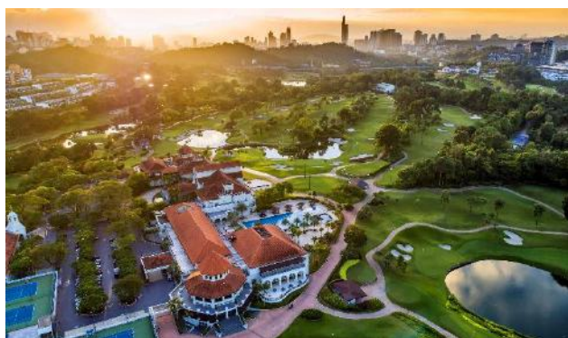
Kuala Lumpur Golf & Country Club, Malaysia
