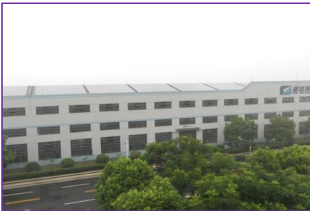
Construction of photovoltaic power station
