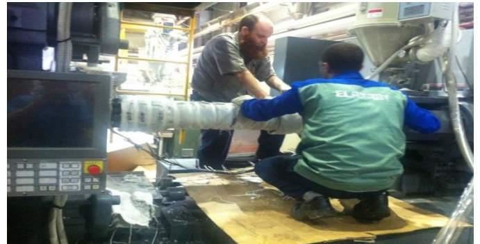
Figure 5: Installed Insulation heater
