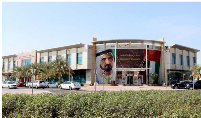
Dubai Municipality – Al Twar Building
