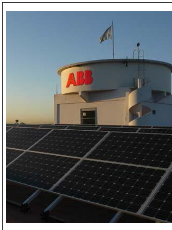
Solar panels in the rooftop of Valentin Alsina facilities
