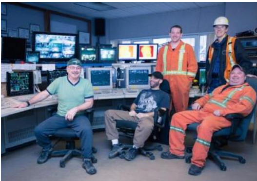
Power & Recovery control room operating Crew
