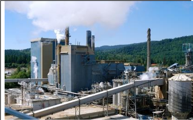
Crofton Mill, Power and Recovery Area
