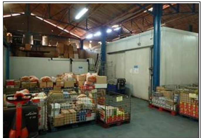
Freezing Chamber and the smaller Cooling Chamber
